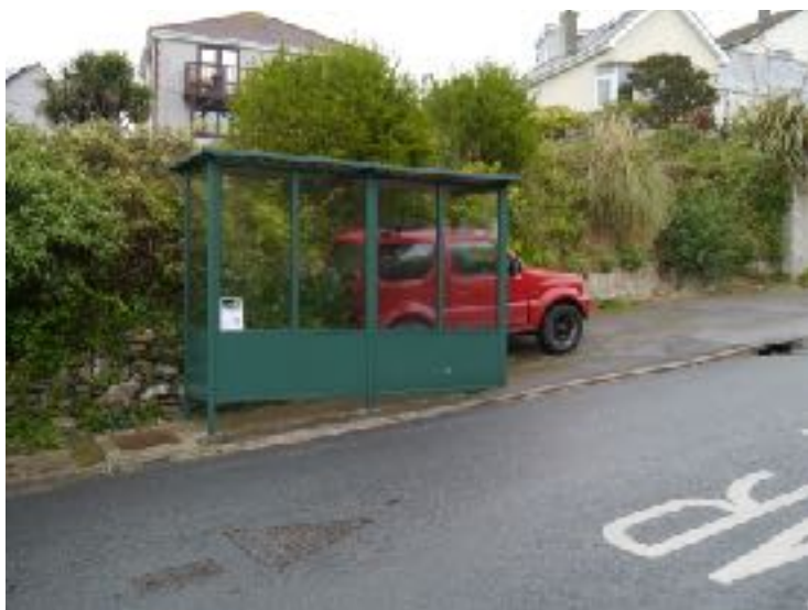
Polruan Shelter Wellside
